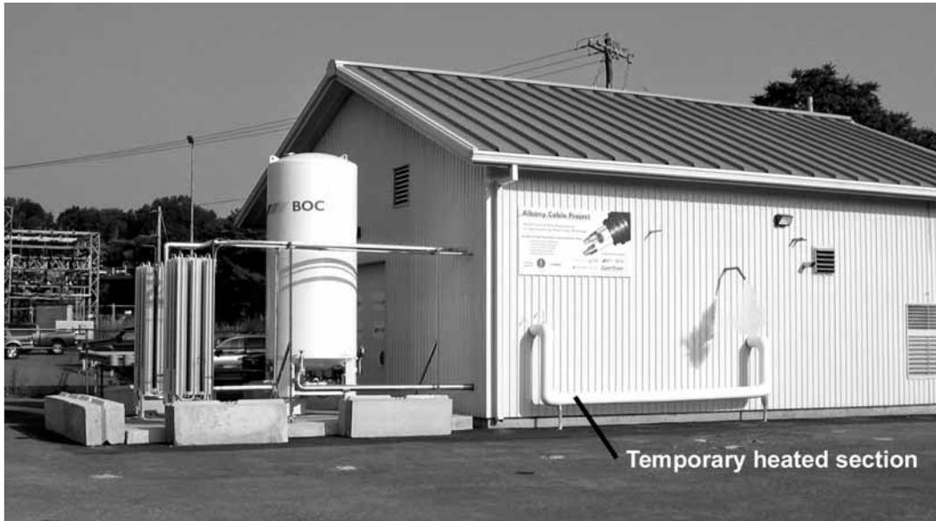
**FIGURE 1.** Albany controls and equipment building with temporary heated section and liquid nitrogen tank.
